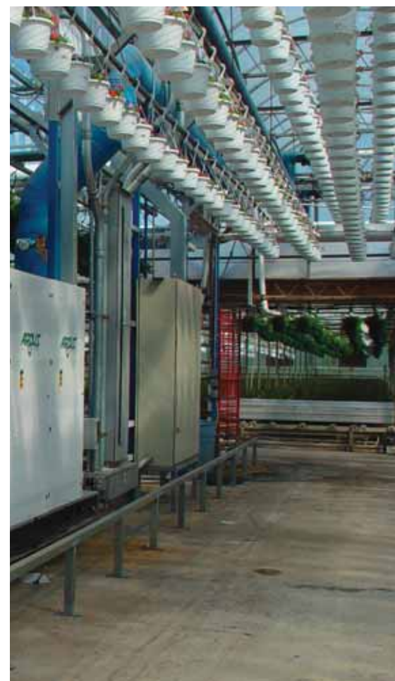
Integrated control systems provide central access and convenient monitoring features.
