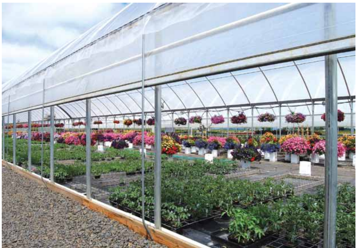
Natural ventilation can be achieved using roof vents, roll-up or drop-down sides, or open end panels.
