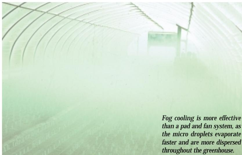
Fog cooling is more effective than a pad and fan system, as the micro droplets evaporate faster and are more dispersed throughout the greenhouse.
