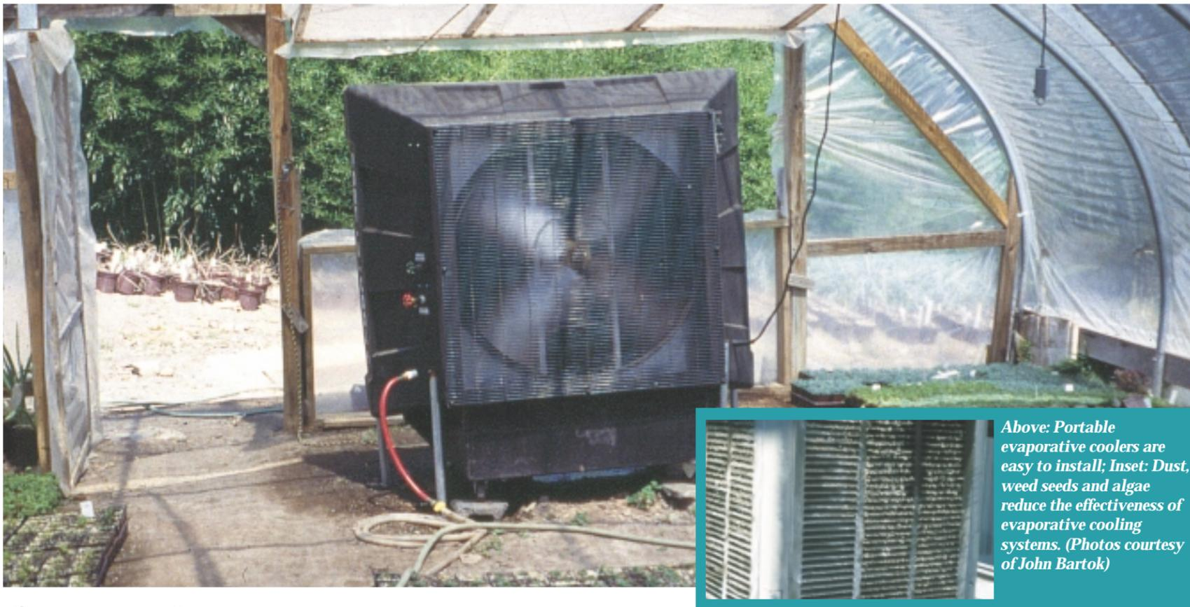
Above: Portable evaporative coolers are easy to install; Inset: Dust, weed seeds and algae reduce the effectiveness of evaporative cooling systems. (Photos courtesy of John Bartok)
