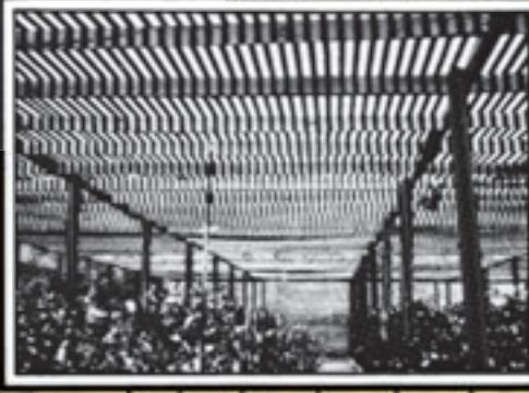
**Woven lath shade and bench fabric** is made of specially selected Grade "A" or better lath  $1\frac{1}{2}$ " space between pickets. The 6' wide material is woven between seven two-wire cables of copper bearing, galvanized wire. The 4' wide is woven between five two-wire cables. Pressure treated, 55% closed, 45% open. These choice pickets are available hot dipped in a red oxide stain, or natural finish; please specify.
