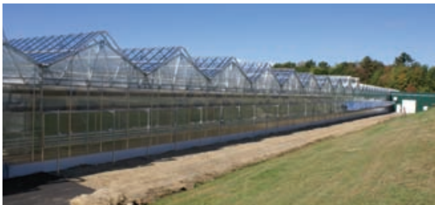
Dual-atrium greenhouses have half the gutters of open-roof structures and fewer working parts.
