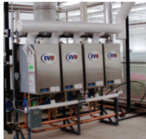
The current drawback to natural-gas heaters is that they are limited in their horsepower capacity, so they are not as cost effective as a lone source of heat for a multiacre facility. (Photo: Hamilton Engineering)
