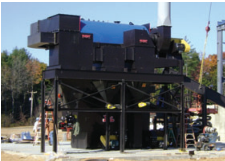
Above: Pleasant View Gardens in Pembroke, N.H., earned a grant for its new biomass boiler system. (Photo: Pleasant View Gardens) Top: With biomass burners, the fuel enters a burn chamber, where air is incorporated with the biomass, which creates a hot, complete burn. (Photo: SAR Biomass)
