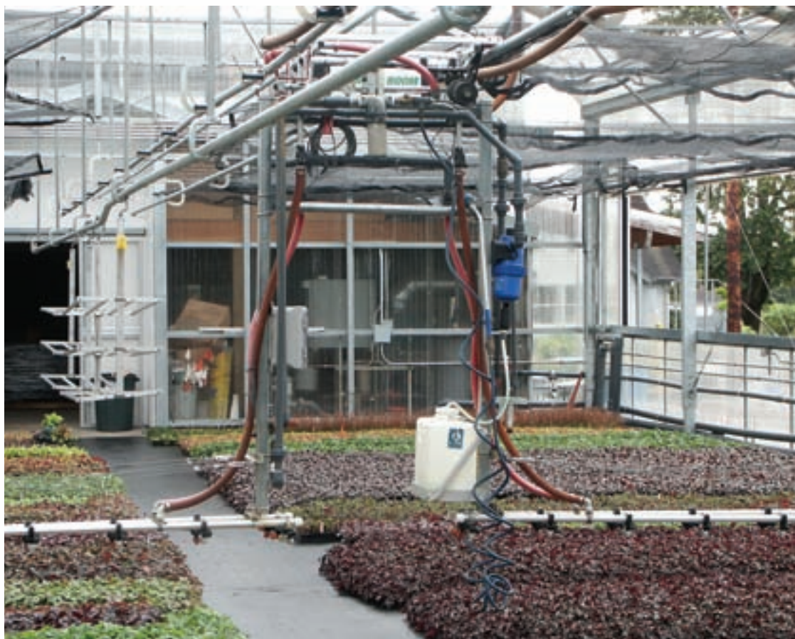
Monorail boom irrigation systems work well in smaller greenhouses. (Photo: Solaris, a Division of McConkey Co.)
