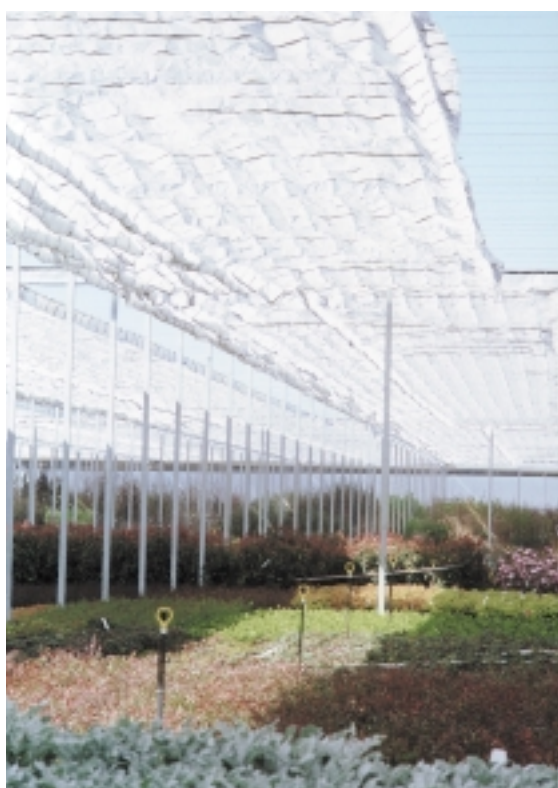
Regardless of type, all open-roof greenhouses provide natural ventilation, better light quality and in-place hardening.
