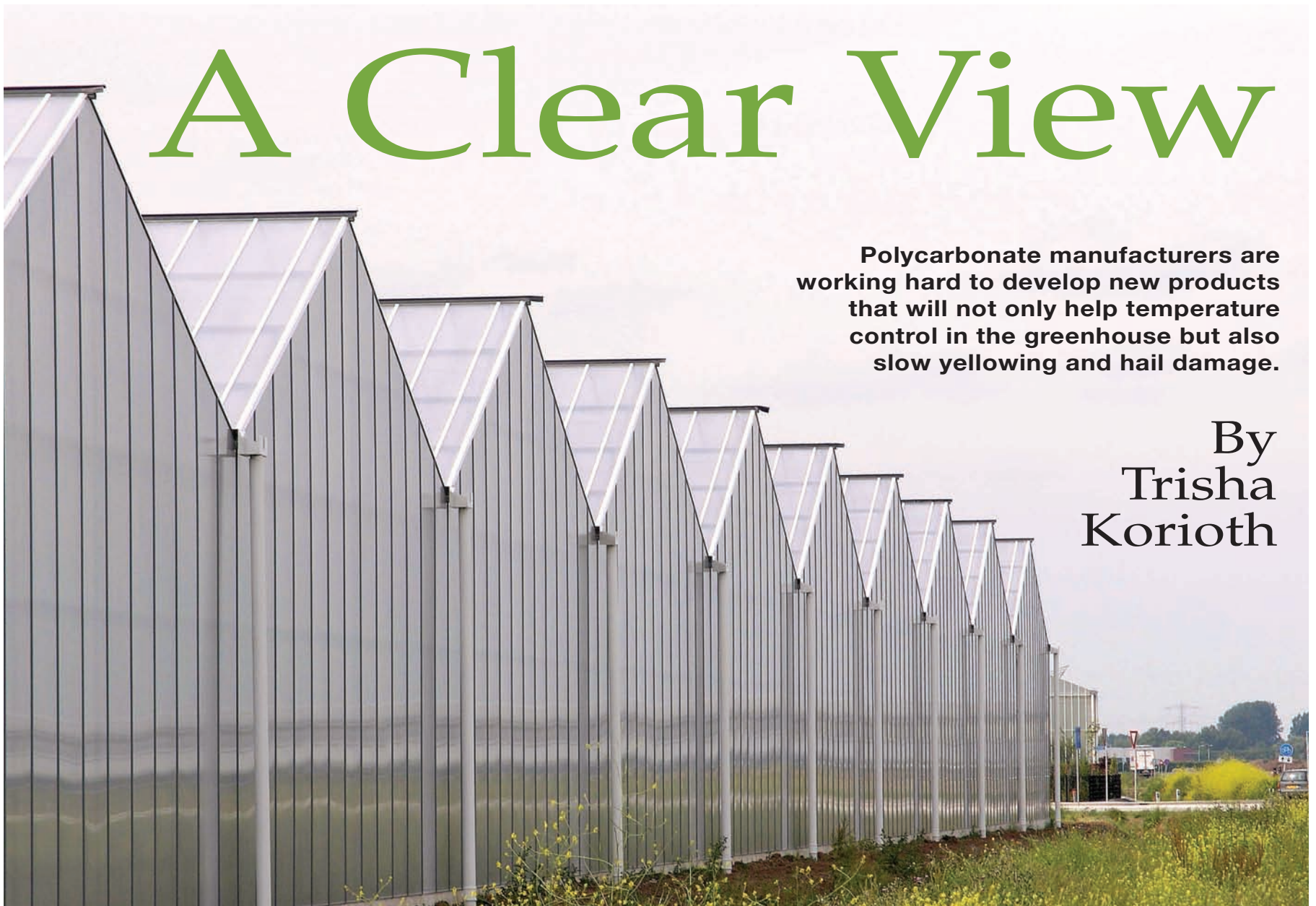
Lexan polycarbonate materials will allow this greenhouse in The Netherlands to produce more energy than it uses, enabling approximately a third of the heat generated to be sold as surplus. (Photos: GE Plastics)
