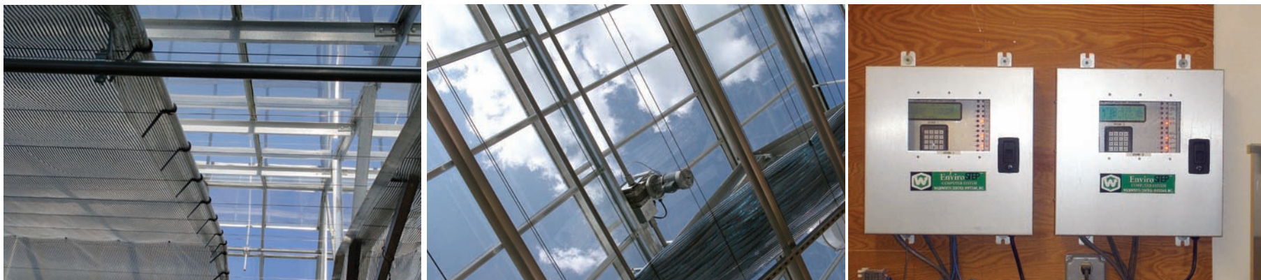
Left: The PowerPull shade system moves over stationary lines. Middle: The PowerPull system fabric is designed to resist UV rays, heat and chemicals. (Photos courtesy of Wadsworth Control Systems) Right: The EnviroSTEP environmental control unit controls the PowerPull curtain and other greenhouse equipment. (Photo courtesy of Barlow Flower Farm)
