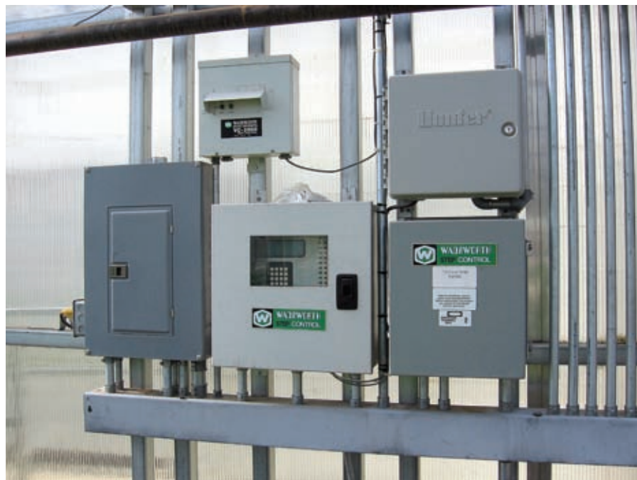
Left: These controls each have their own contactor panel, power pull energy curtain control box and four vent control boxes. This is a complete system. Right: This is an EnviroSTEP control, contactor panel and vent control box at a garden center.
