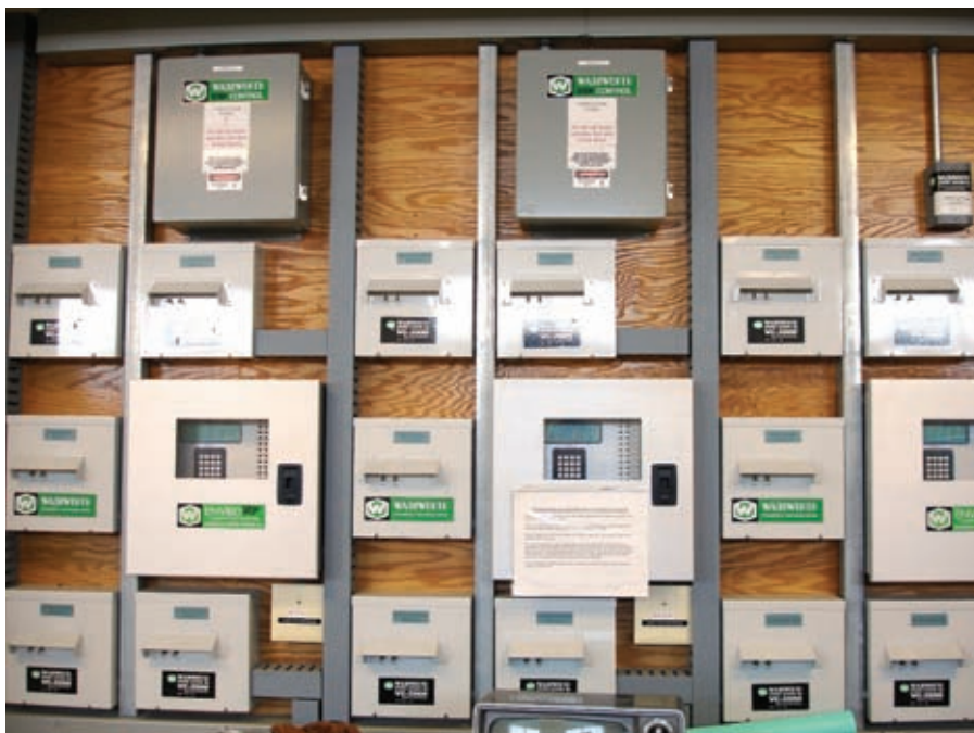
Left: These controls each have their own contactor panel, power pull energy curtain control box and four vent control boxes. This is a complete system. Right: This is an EnviroSTEP control, contactor panel and vent control box at a garden center.
