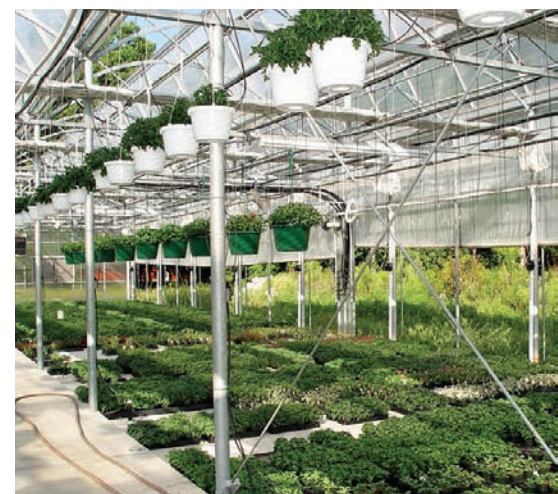
Install roll-up greenhouse sides for more efficient cooling. (Photo: Lawrence Martin)
