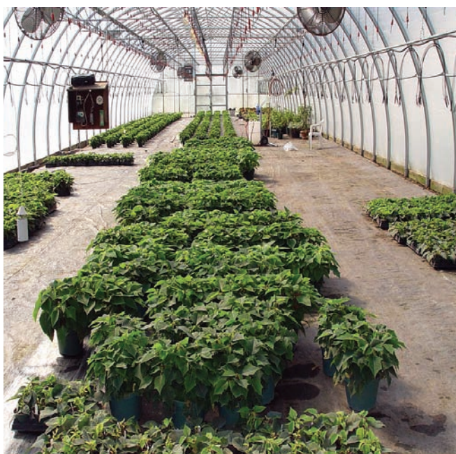
A single layer of film over glass can reduce annual heating costs 5-50 percent, whereas a double (inflated) layer can reduce costs 40-60 percent. (Photo: Lawrence Martin)
