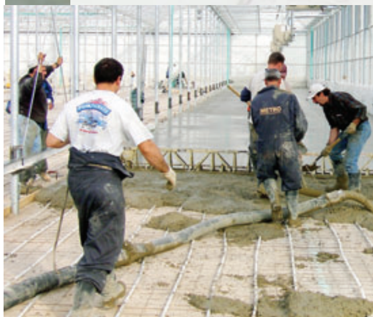
Top: Flood floors use in-floor heating, creating a microclimate that stimulates root growth. Bottom: When designing a flood floor, the first step is to decide which style works best for your greenhouse.
