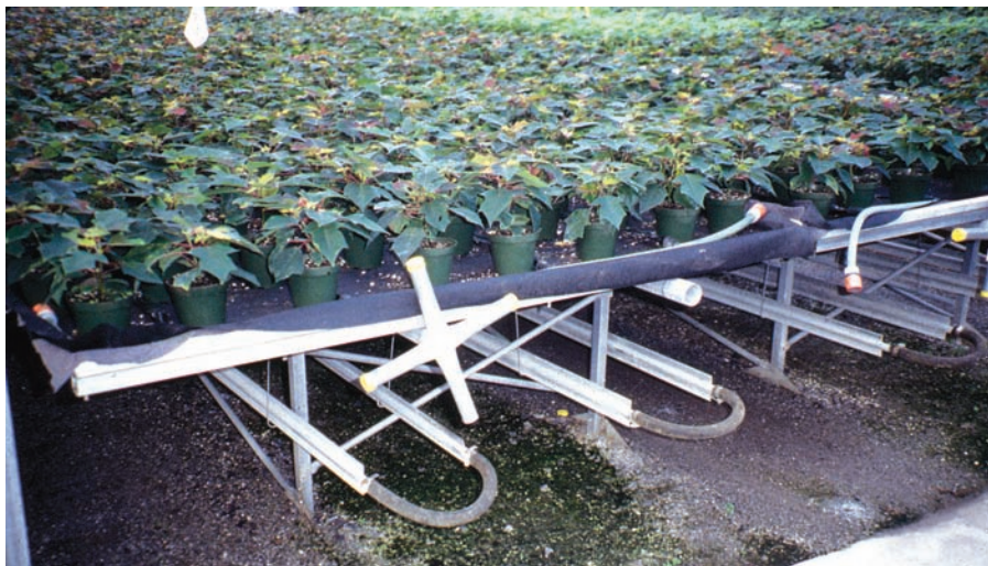
Left: Low-output fin radiation is easy to install and out of the way of plant handling. Rubber tubing connects the separate runs of aluminum pipe. Right: A plastic weed mat material attached to the bench sides contains the heat underneath the bench and allows the air temperature to remain cooler.
