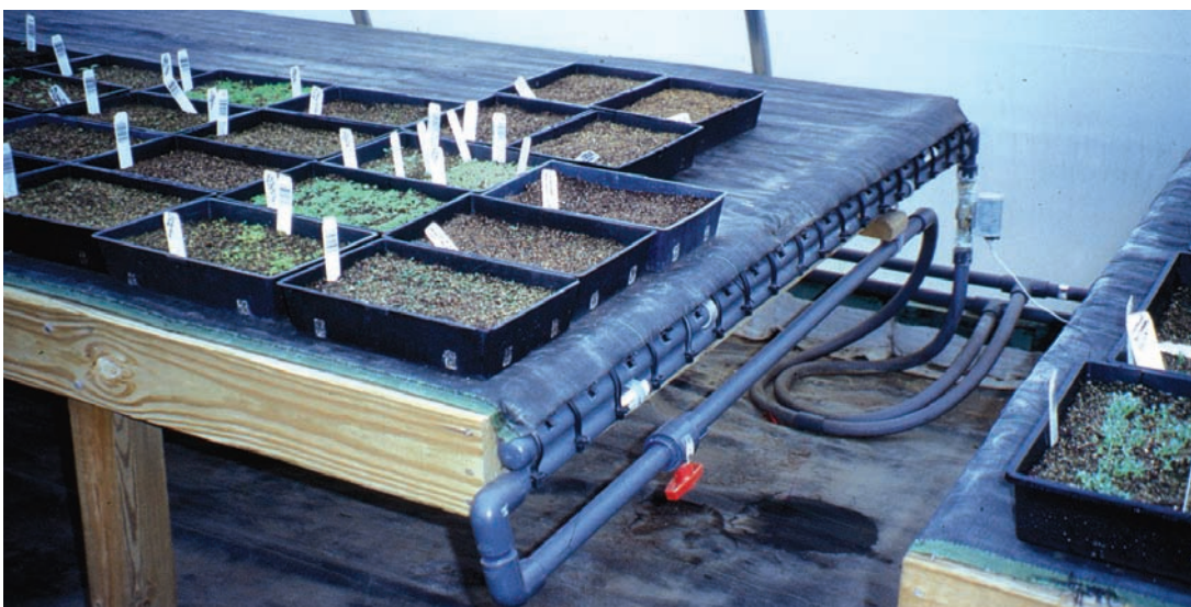
Rubber tubing and PVC pipe are used to supply this flat-top root zone heat mat. PVC pipe can handle up to 130° F water without sagging.
