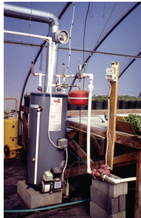
Top: A small boiler is a good source of hot water for the root zone heating system. Different temperature zones are supplied water from circulating pumps and controlled by remote bulb thermostats. Bottom: For small bench areas up to 2,000 sq.ft., a domestic hot water heater works well. The thermostat on this oil-fired heater is set to the desired 100-120° F water temperature. (Photos: John Bartok, Jr.)
