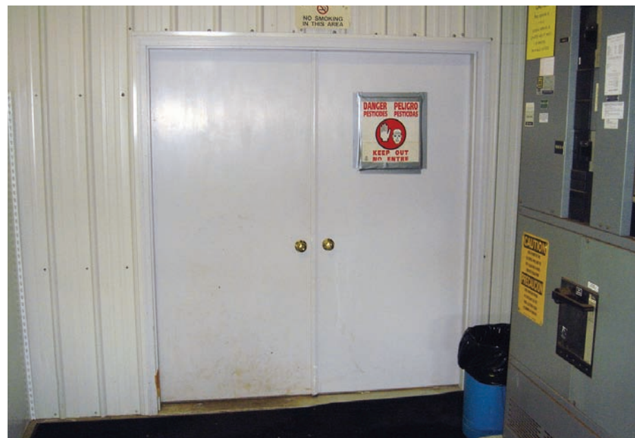
Make sure pesticide storage is properly signed and locked.
