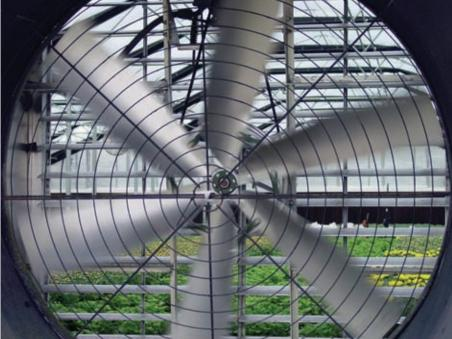
Left: Keeping grass and other elements clear of exhaust fans will increase the amount of air a fan is able to pull out of the greenhouse. Right: Dirty blades can reduce the amount of airflow on a single fan by as much as 20-40 percent without proper cleaning.
