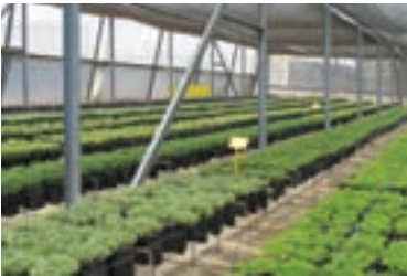
Greenhouses are full-metal construction with wire benching and concrete floors. No wood is allowed in the structure for cleanliness reasons.
