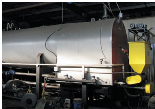
Van Wingerden purchased a wood pellet boiler to create an alternative energy source to fossil fuel, reducing dependence and saving money at the same time.
