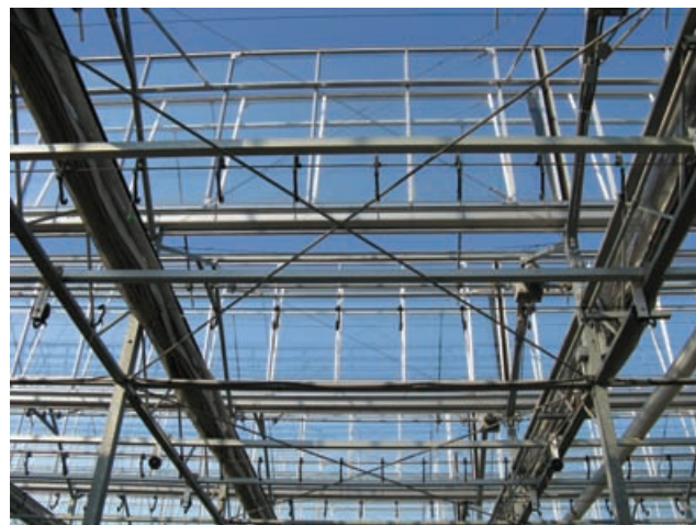
Open-roof ranges, equipped with shade and energy curtains, provide ideal environments for plant growth and aid in fuel savings.
