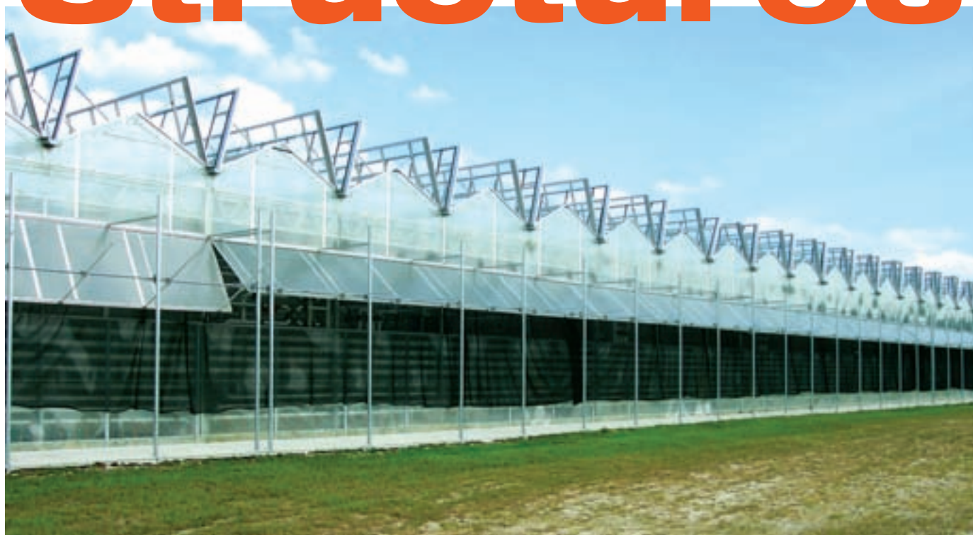
Manufacturers feel open-roof greenhouses — both 100-percent and partially open — are likely to continue being popular. (Photo: Nexus Greenhouse Corporation)
