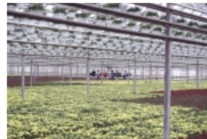
Flood floor system maximizes efficiency in a high greenhouse space.
