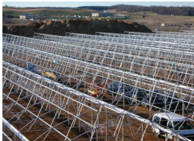
Plant Marketing, Eau Claire, Wis., recently built a 5½-acre naturally ventilated range. This new range has helped Plant Marketing increase production efficiency and its ability to deliver product throughout the Midwest. (Photo: Nexus Corp.)
