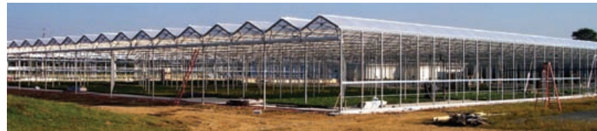
To control their energy costs, many growers are looking for a greenhouse like this one under construction that will let sunshine in and excess heat out. (Photo: X.S. Smith)
