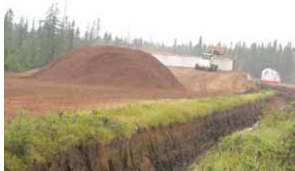
Figure 2. The drainage ditch (foreground) reveals, how thick the layers of peat are in this particular bog.
