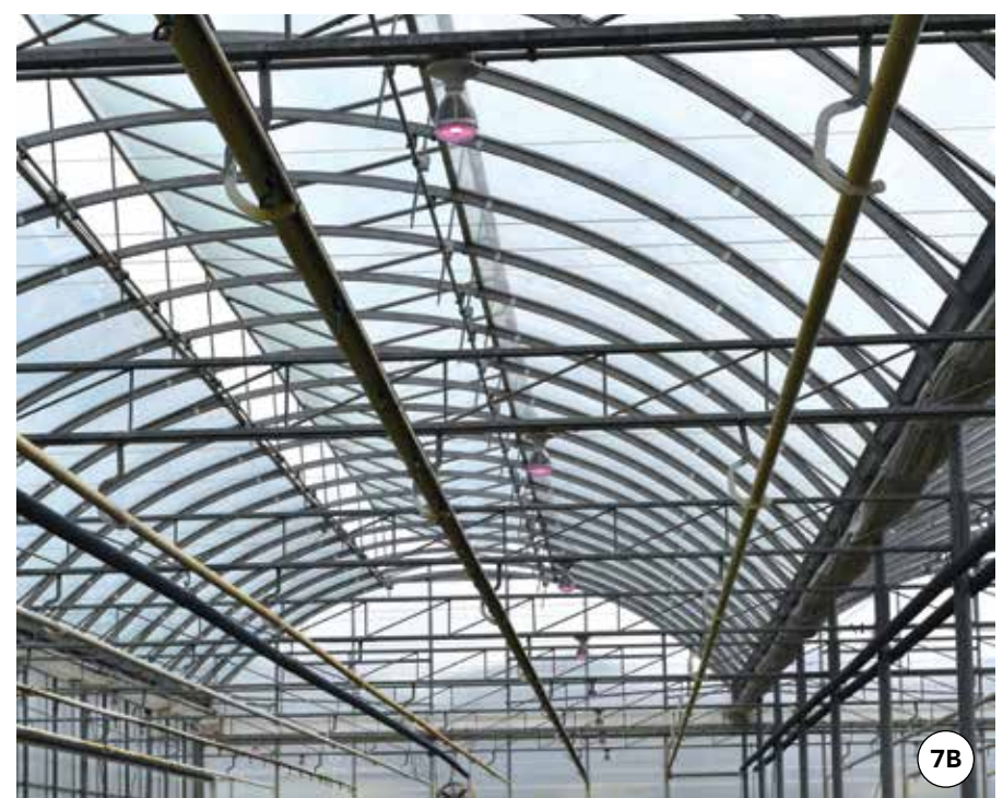
Figure 7A) Installations of Ventis Philips GreenPower Flowering LED Flowering Lamps and 7B) Ventis Total Grow Night & Day Management Light LED used for photoperiodic lighting at a commercial greenhouse.
