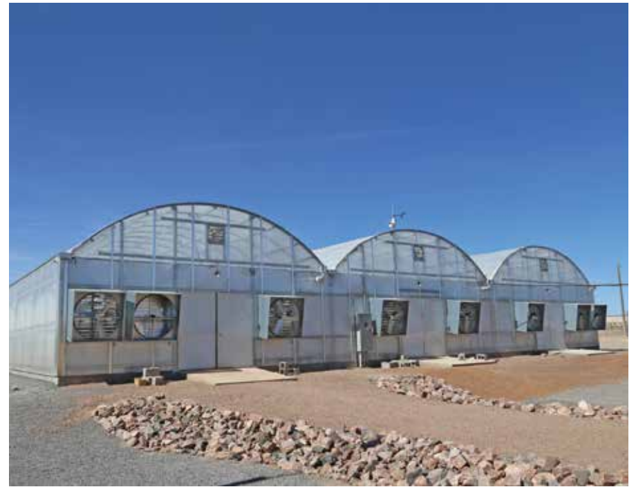
Designing a sturdy greenhouse that is also tailored to a specific operation is a unique blend of foundation, frame and covering.
