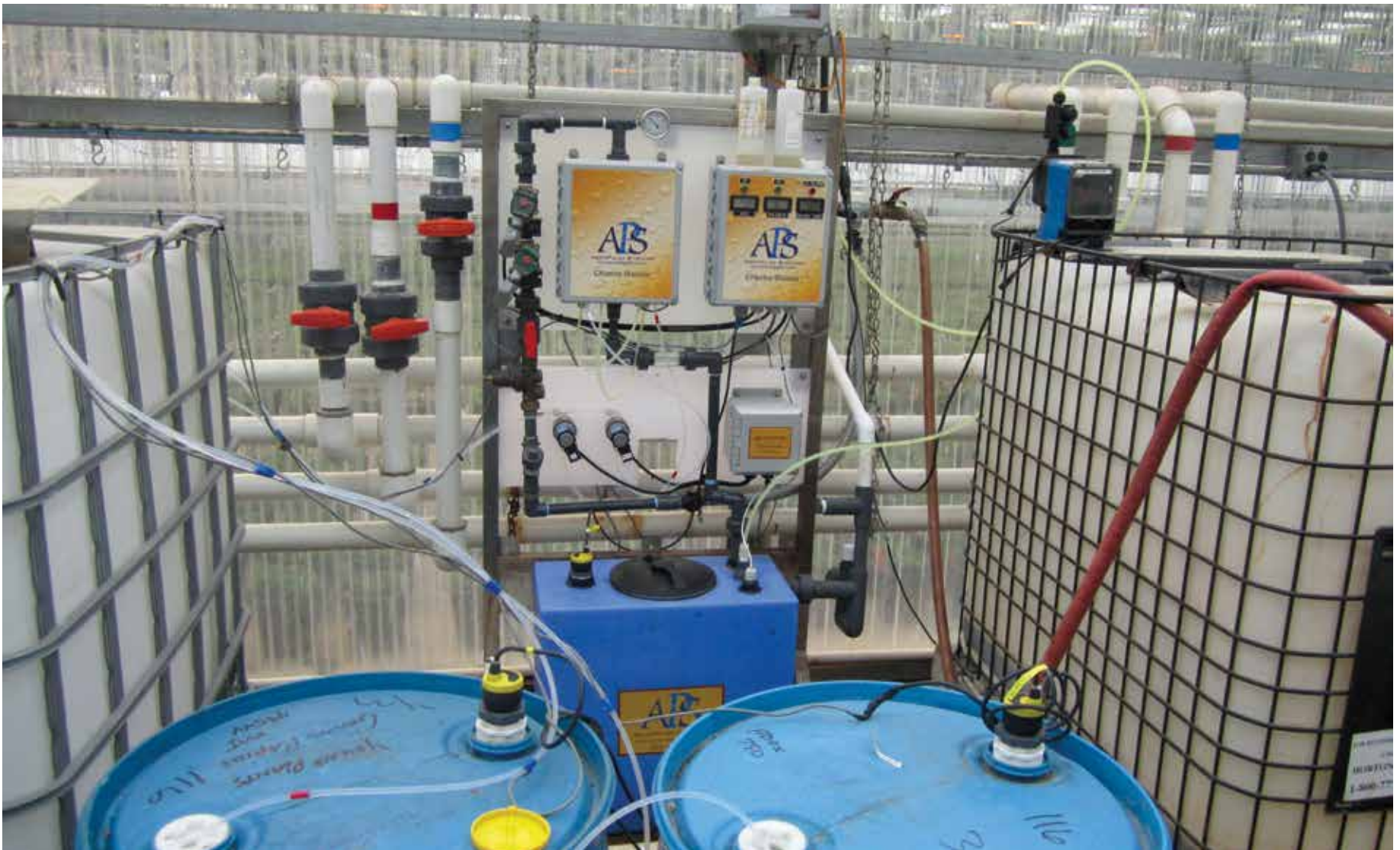
Figure 4. Chlorine dioxide two-tank system.
