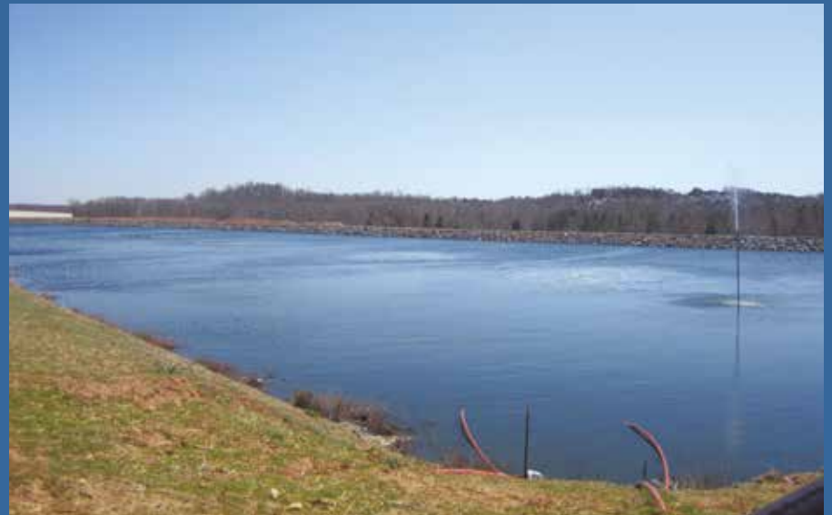
Figure 1. Irrigation pond in which irrigation runoff is collected.
