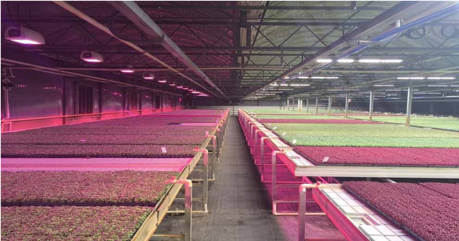
Figure 2. The spectrum (i.e., color) of light emitted from a horticulture lighting solution has a significant impact on both energy efficiency and overall plant growth and development. While red and blue light is more energy efficient to produce, a broad spectrum will target more photoreceptors for improved cultivation and improve visual acuity to scout for pests and diseases.
