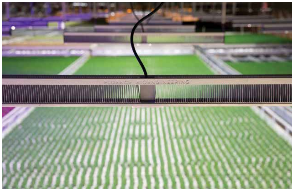
Figure 3. The form factor of a horticulture lighting solution is critical to avoid blocking ambient light from your crops.
