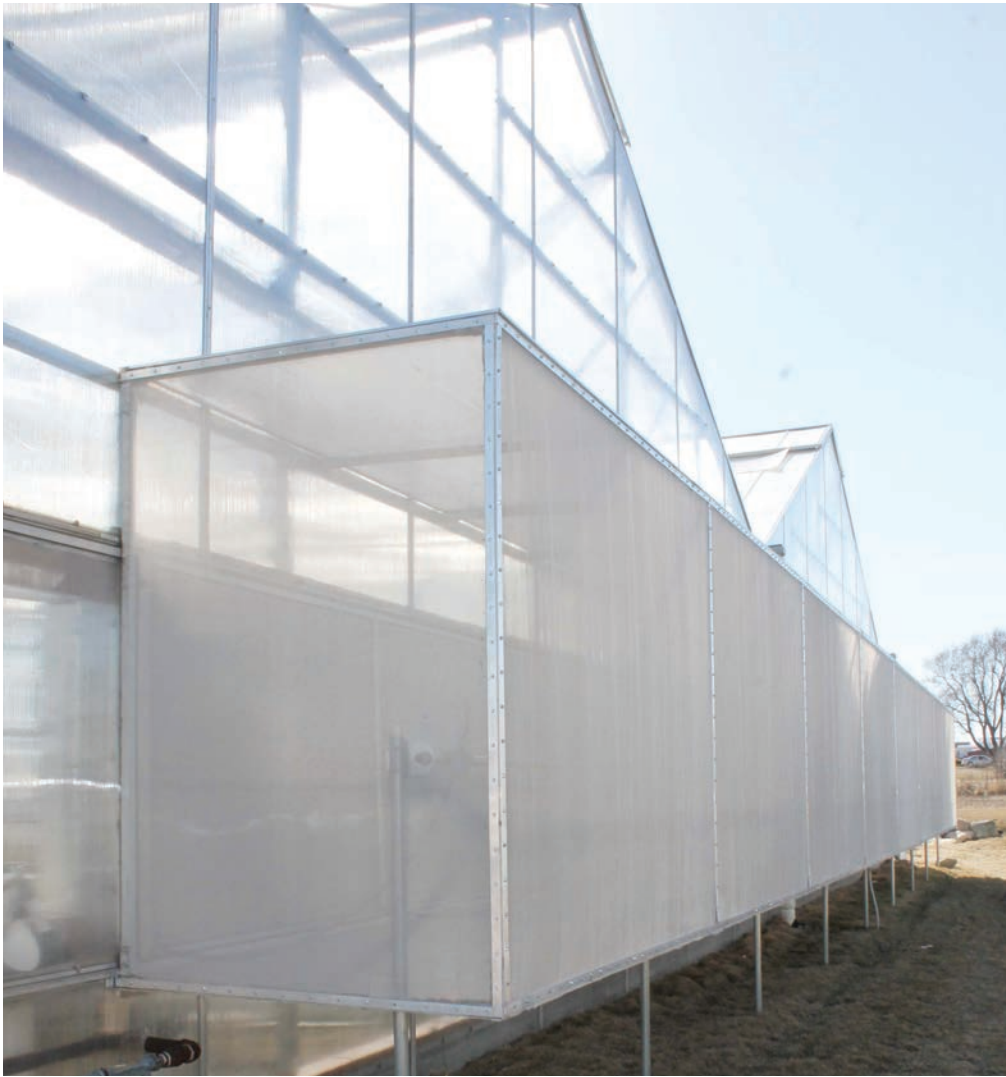
Installing screens helps prevent insects from entering the greenhouse and damaging plants.
