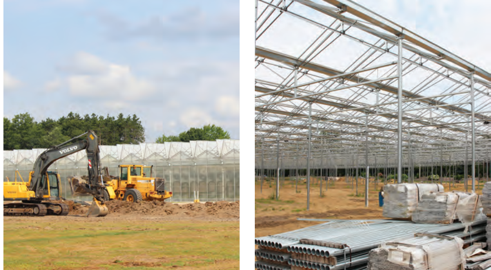
The team at Spring Meadow is constantly building new greenhouses to meet the growing needs of the company's customers.
