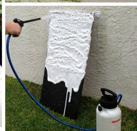
Pair chemical cleaners with a foamer to increase wet contact time and ensure all areas have been treated.
