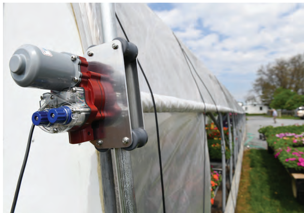
Automated roll up curtain system.
