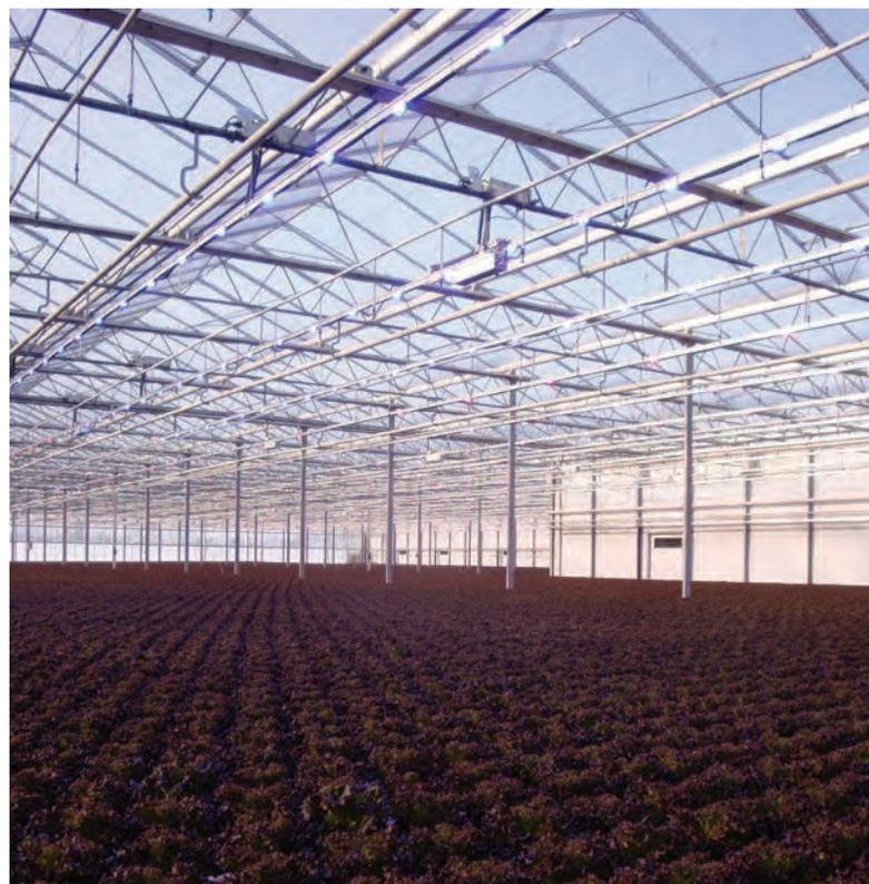
**Figure 1.** The design, infrastructure, selection of glazing materials, and positioning of equipment are among the factors that influence transmission of sunlight to crops and thus the daily light integral.
