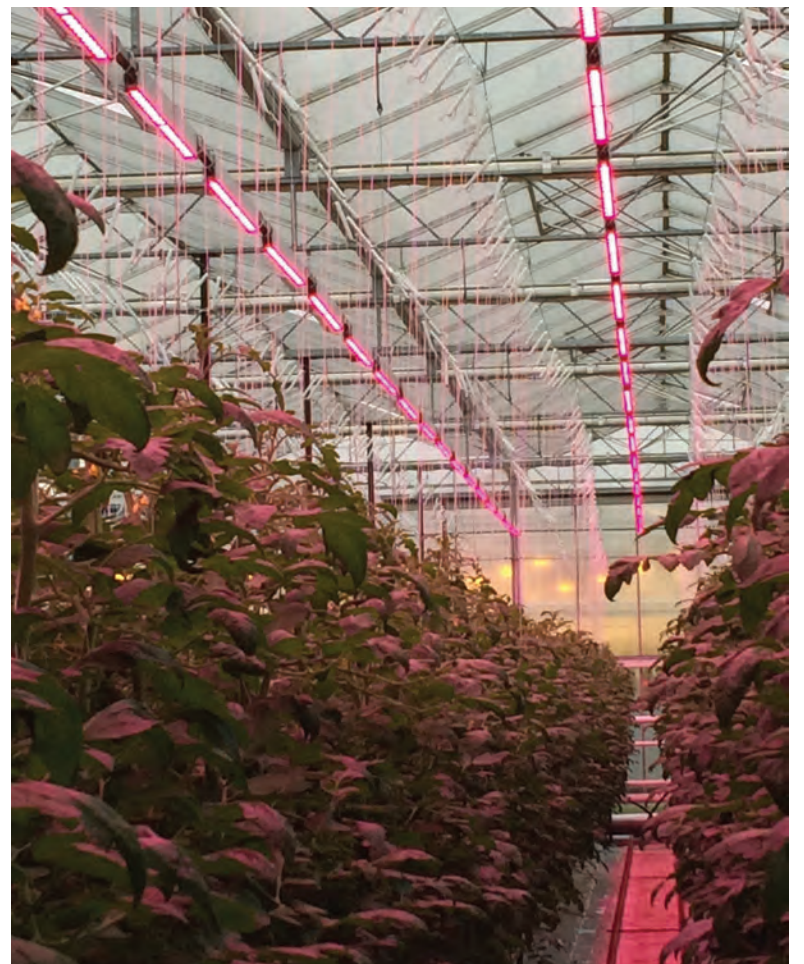
Figure 1. Because red photons have less energy than those with shorter wavelengths, the most effective LED fixtures usually emit at least 90% red light.
