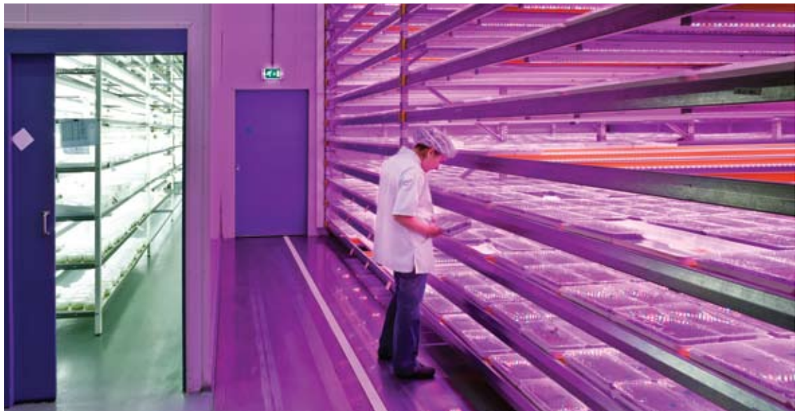
A production center where you can see the new installation with LED production modules as well as the old fluorescent lighting installation
